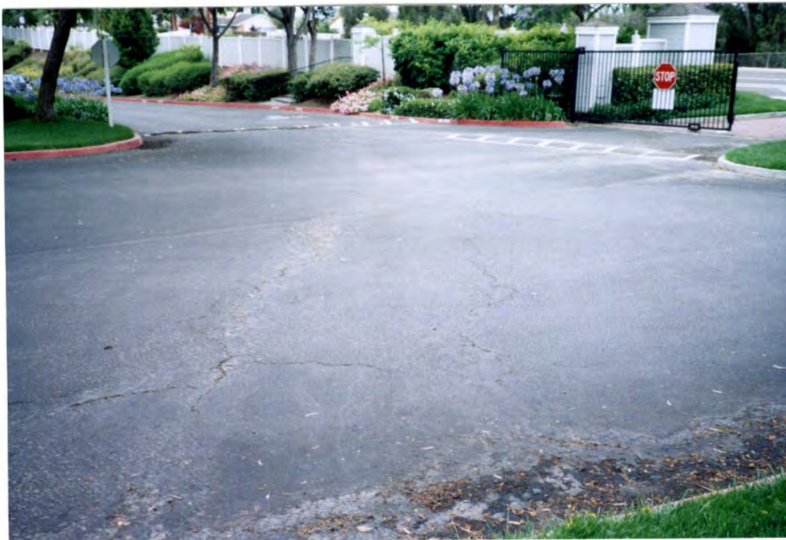
PAVING: Asphalt Slurry / Overlay
