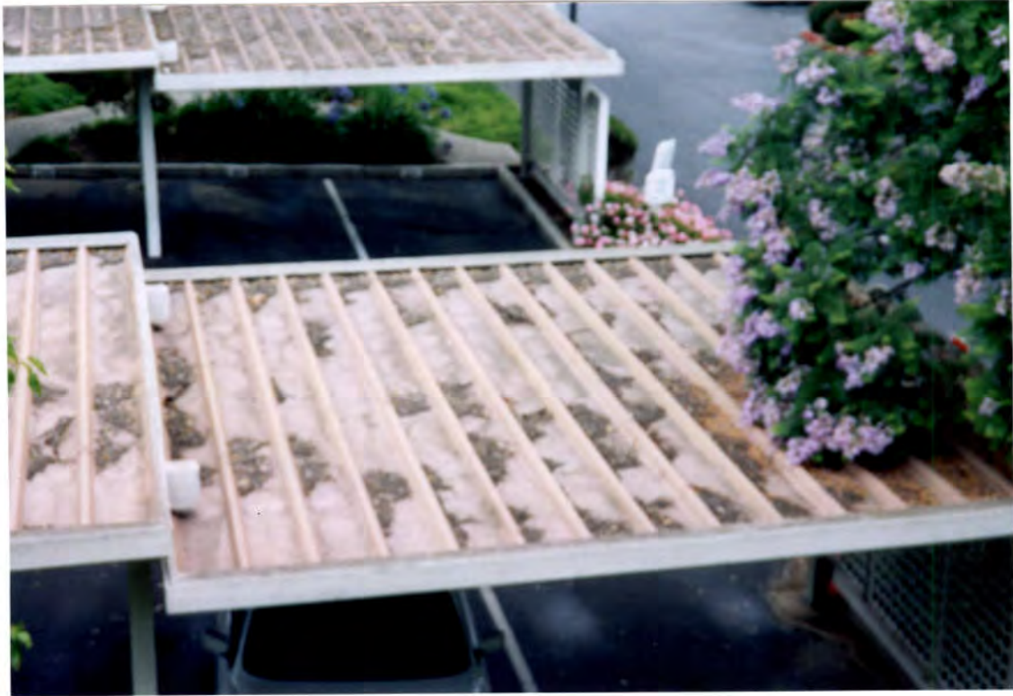
ROOFING: Carport Metal
