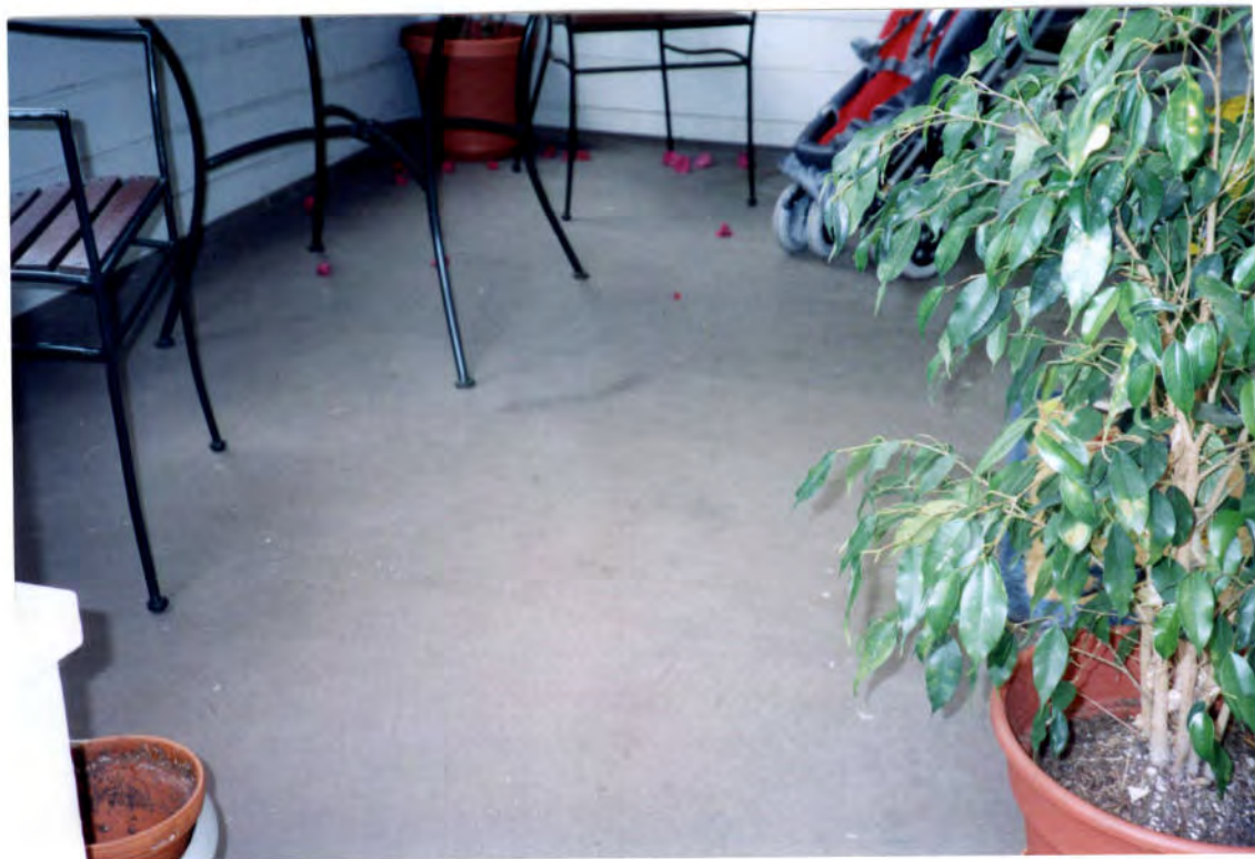
DECKING: Stair Landing ReSeal / ReSurface
