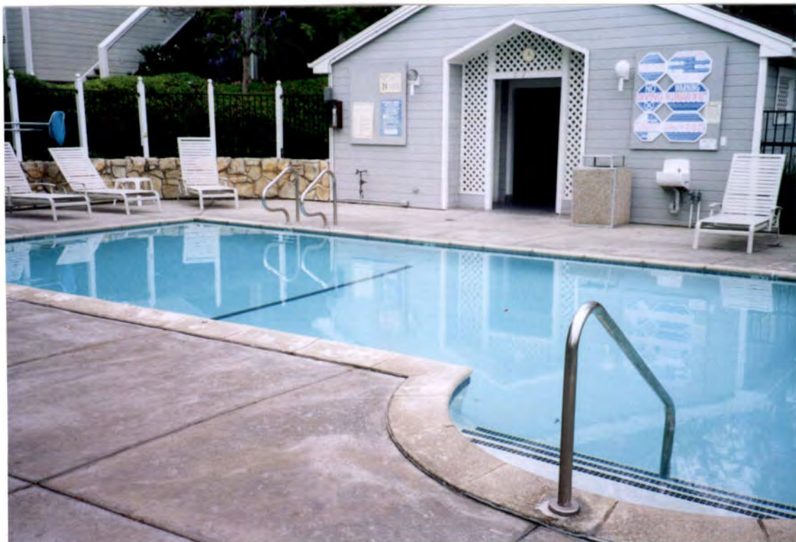
POOL AREA: Pool Replaster
