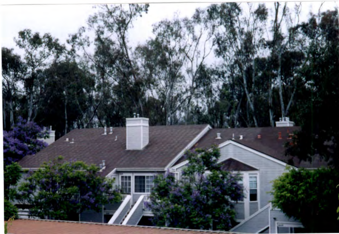
ROOFING: Composition Shingle
