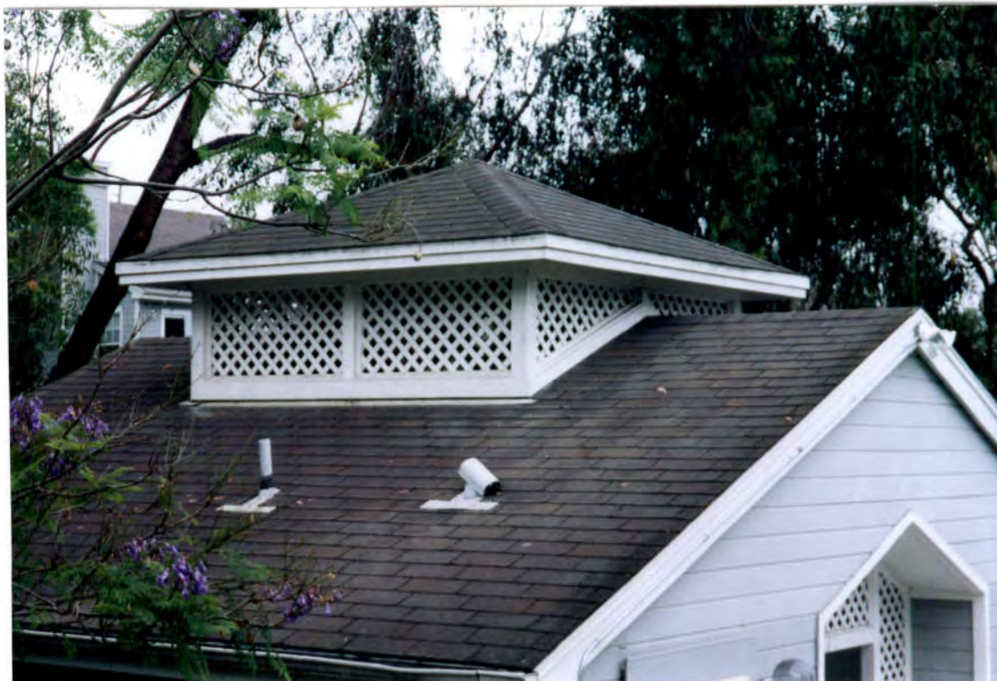
ROOFING: Composition Shingle
