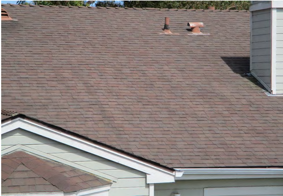
ROOFING: Composition Shingle
