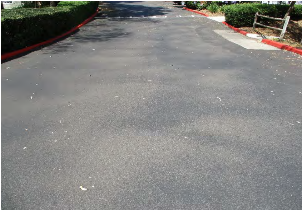
PAVING: Asphalt Slurry / Repair / Overlay
