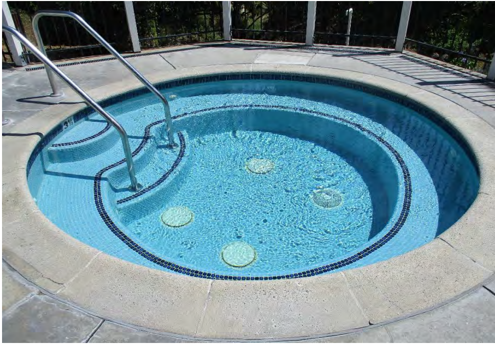
POOL AREA: Spa ReTile
