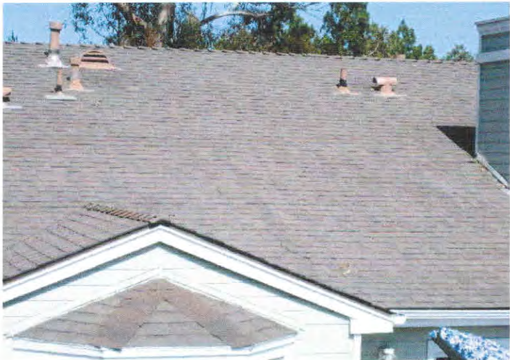
ROOFING: Composition Shingle
