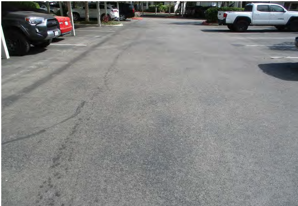
PAVING: Asphalt Seal & Repair / Overlay
