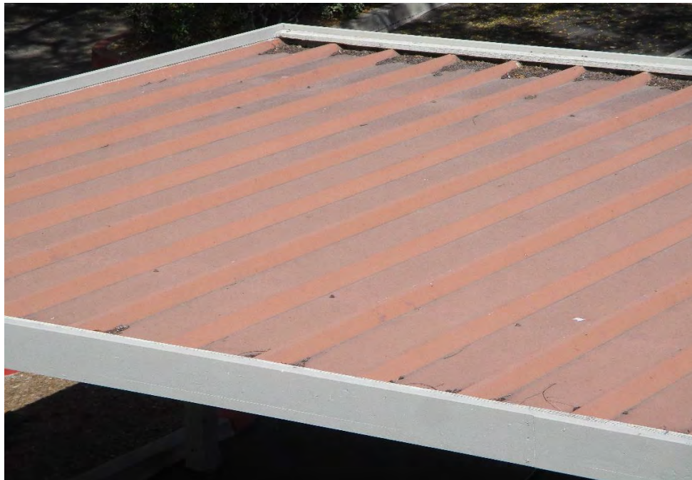
ROOFING: Metal Carports
