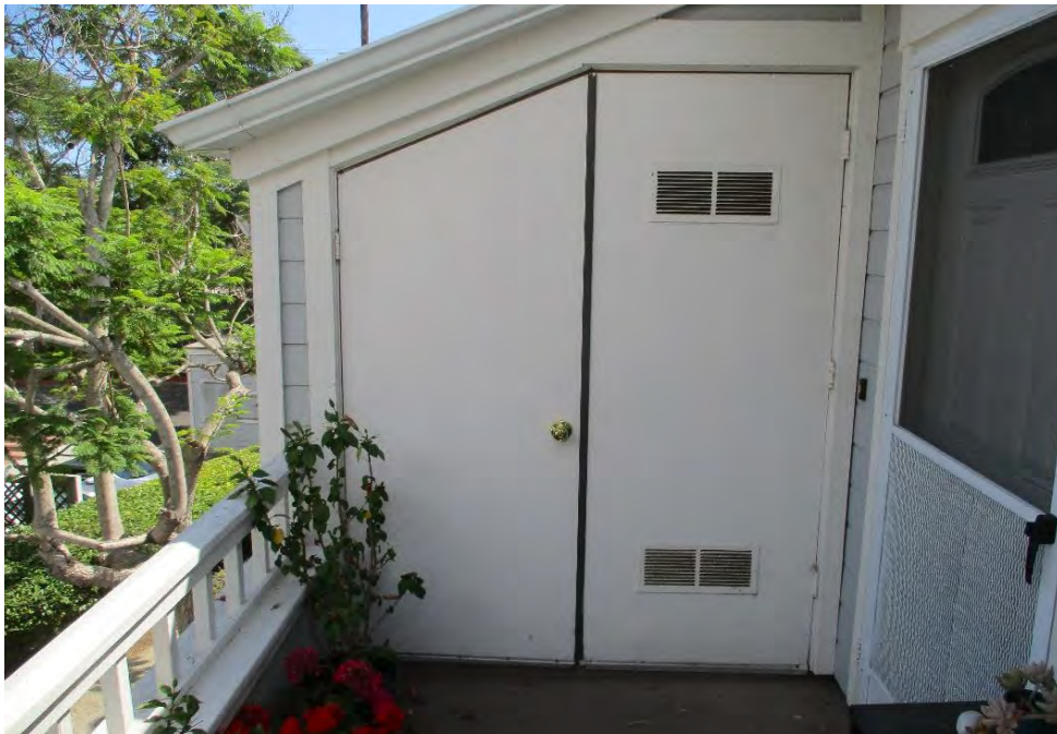
PRIVACY / FENCING: Patio Utility Doors
