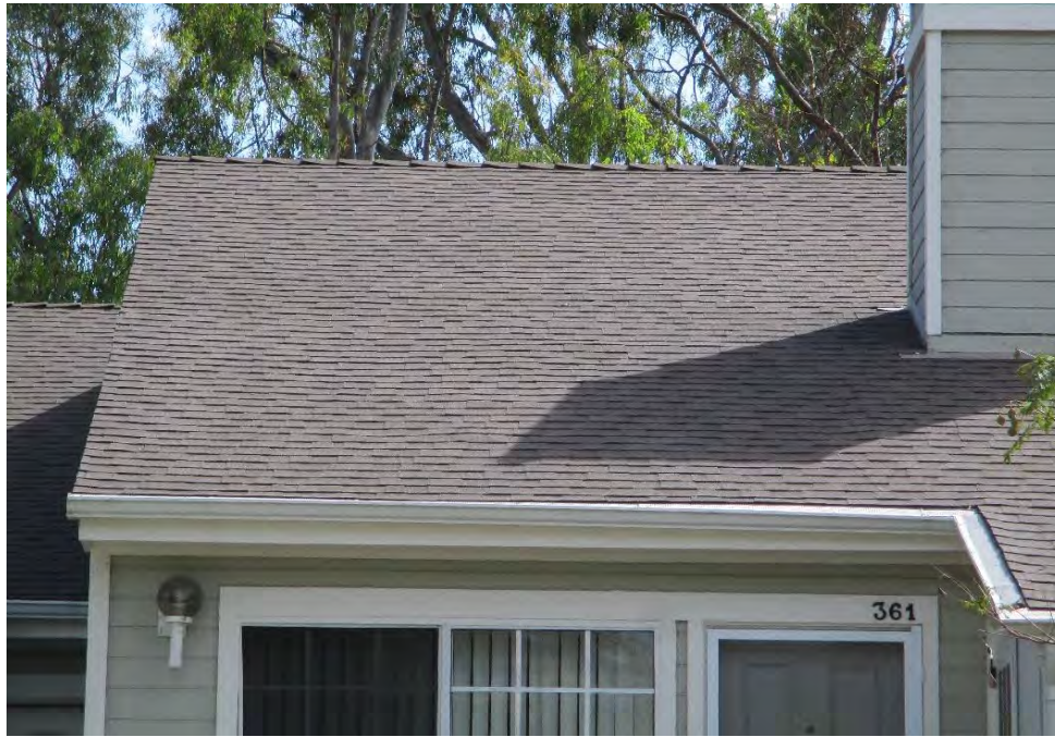
ROOFING: Composition Shingle
