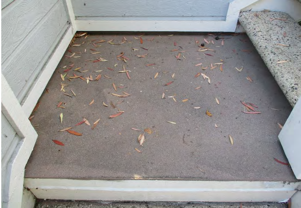
DECKING: Stair Landing ReSeal / ReSurface
