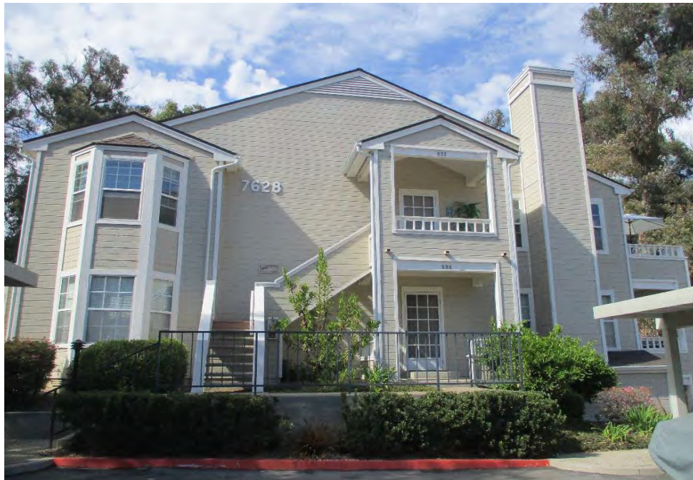
PAINTING: Wood Siding / Wood & Metal Trim / DryRot Repairs
