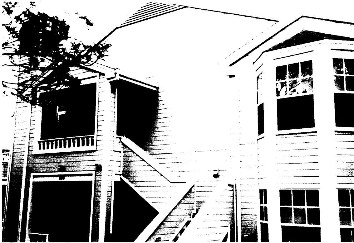
PAINTING: Wood Siding / Trim
