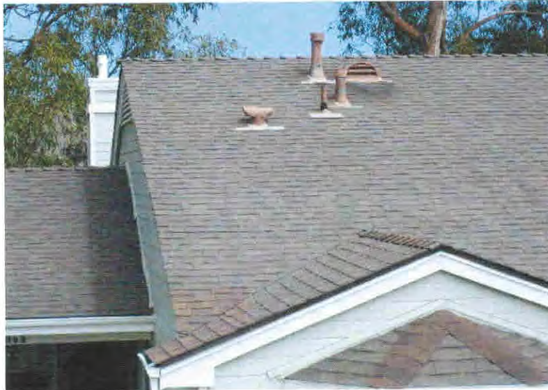
ROOFING: Composition Shingle
