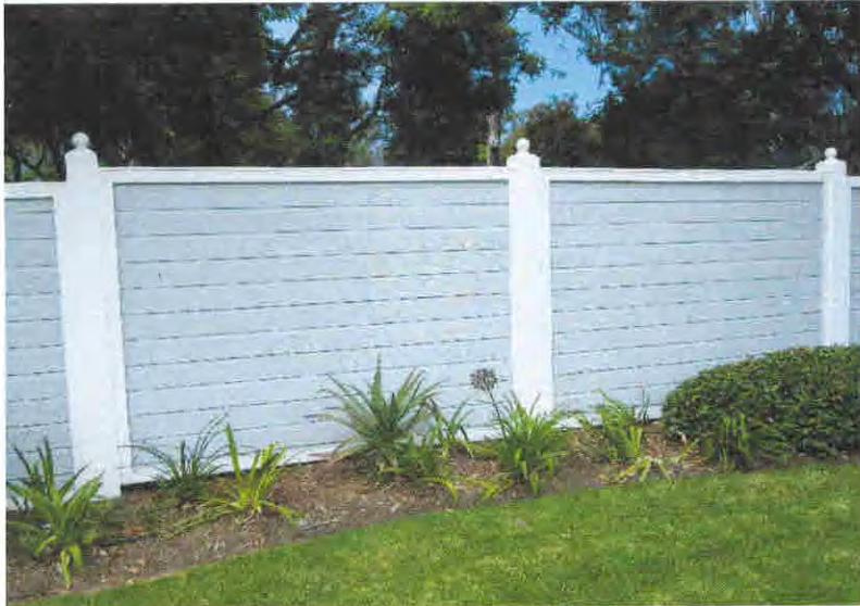
PRIVACY/FENCING: Front Wood Fence
