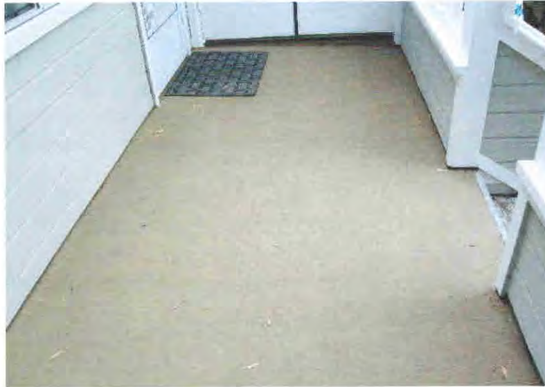
DECKING: Stair Landing ReSeal / ReSurface
